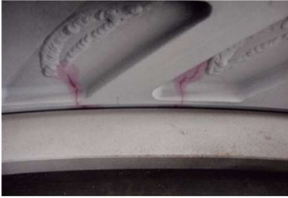
MS5001 Blade Crack Inspection
