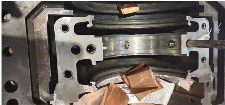
Pre-Repair Condition – Bearing Housing
