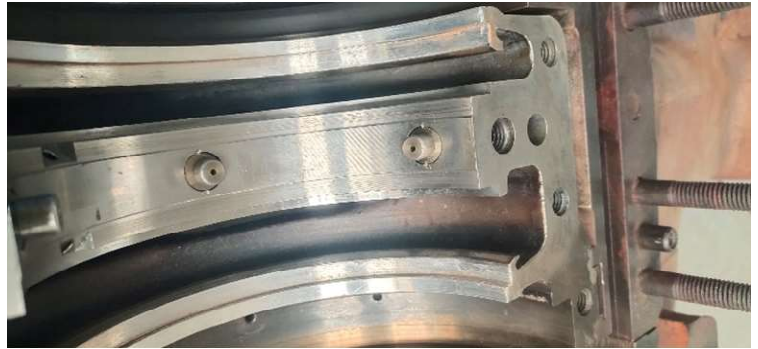
Post-Repair Condition – Bearing Housing
